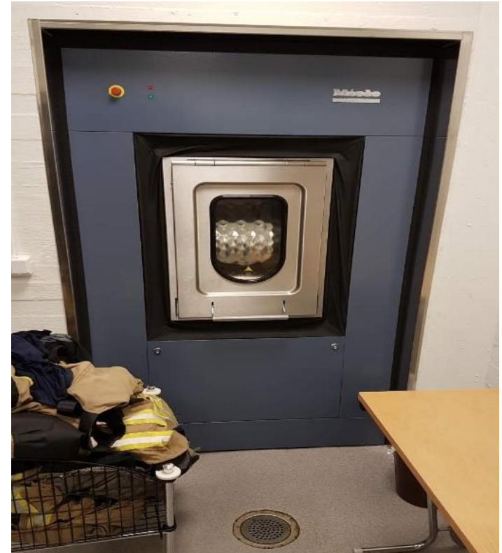
Picture 11 and 12. Examples of barrier washing machines that can be programmed with the Lejon Kemi washing program for breathing masks with or without disinfection steps.
