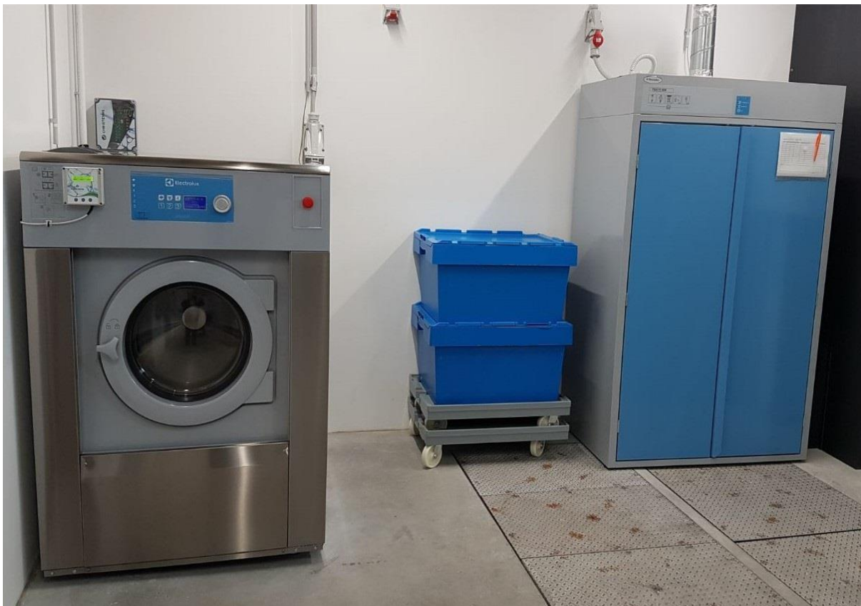
Photo 1. Laundry room at fire station with washing machine and drying cabinet for emergency suits and breathing masks.
